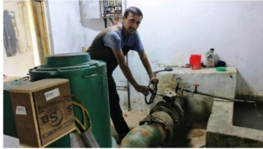
Fig. 3. Operating controlling the water flow to the turbine through the butterfly valve (Source: Surendra Pandit).
